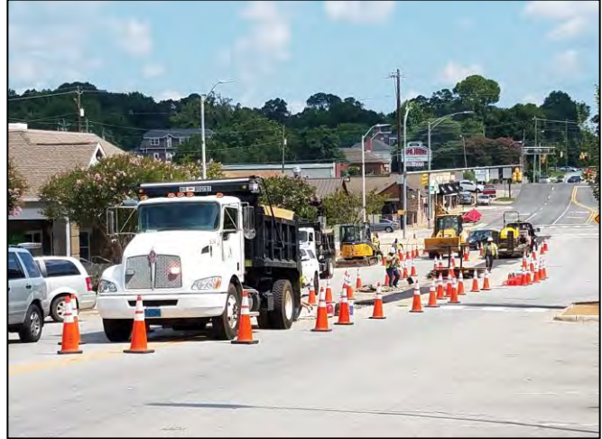
Sewer Main Replacement Project on College Street
