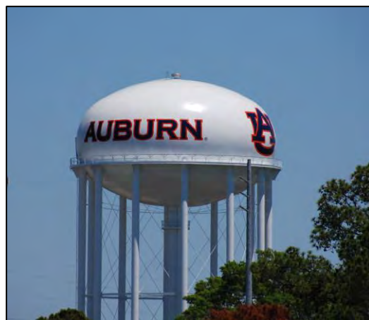
Glenn Avenue Water Tank
