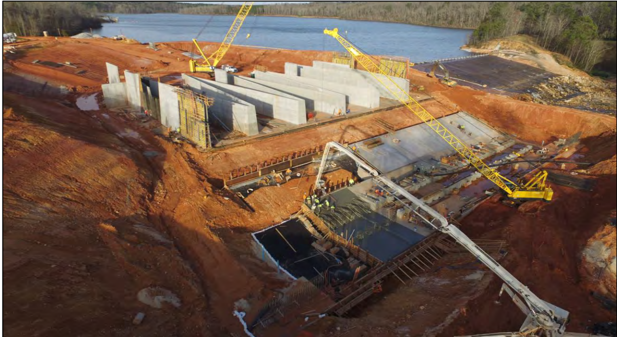
Lake Ogletree Spillway Construction
