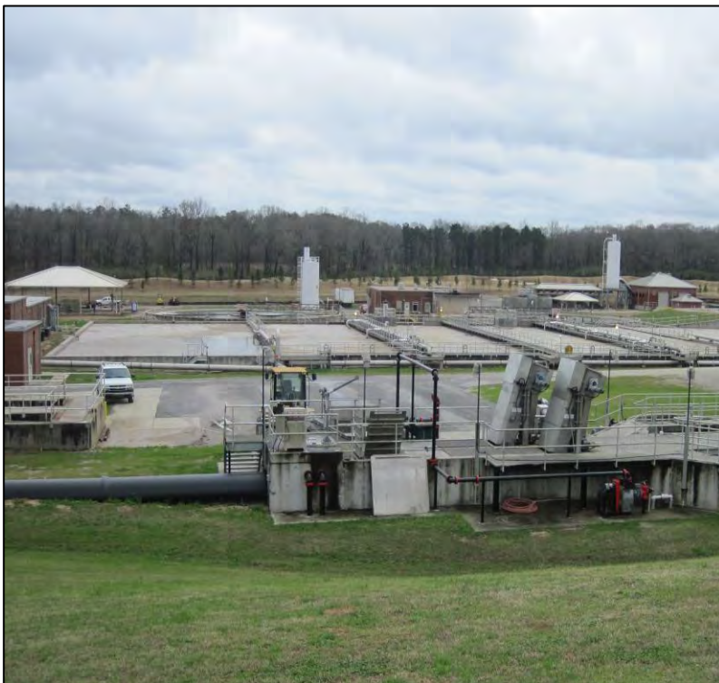
H.C. Morgan Water Pollution Control Facility
